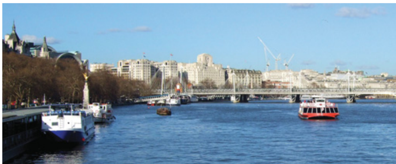
Hungerford Bridge, London.
